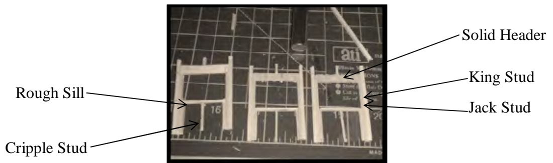
Photo 8: Rough opening of windows and elements. Photo Courtesy of Eman Al-Somali
